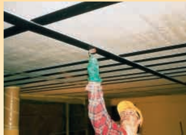
Strengthening of the reinforced concrete slab with the Sika® CarboDur® Plate System (Sikadur-30 adhesive and Sika® CarboDur® plates)
